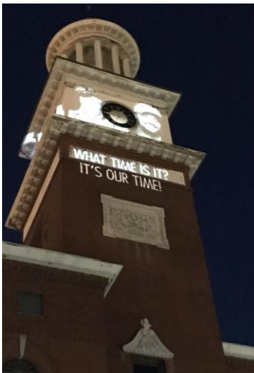
Image of the Clock Tower during the It's Our Time Open House. Projections were provided by Lumenarrt.
